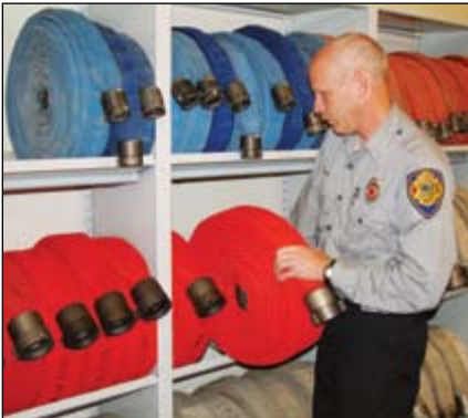
Fire Hose Rack
